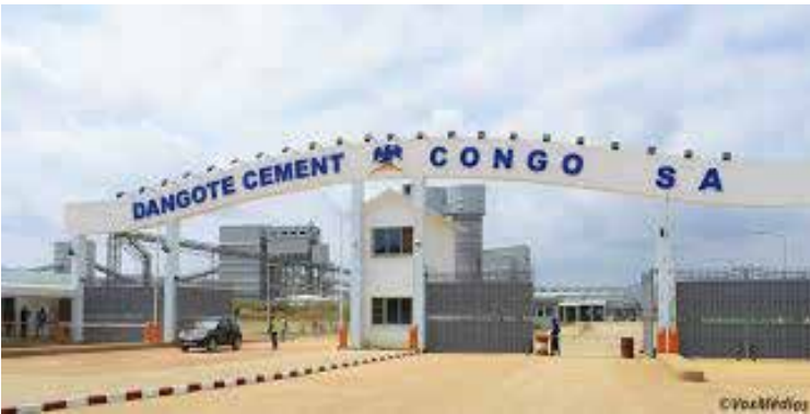
DANGOTE CEMENT CONGO
